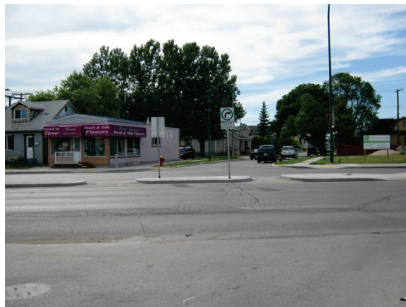
A median refuge helps cyclists cross McPhillips at Pritchard, but cyclists have no way of stopping traffic on this high volume street
