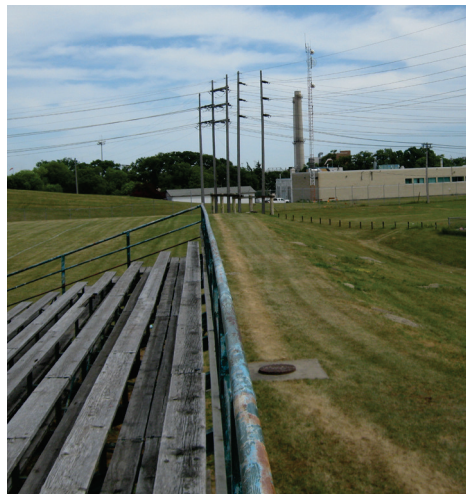
Looking east towards the McPhillips Pumping Station from the grandstand on McPhillips Athletics Grounds
